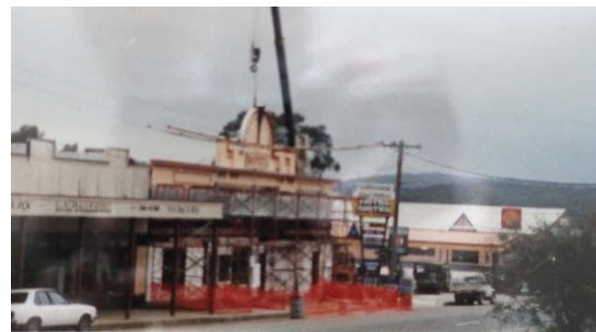
Lifting of new parapet onto the hotel (early 1990s) (Source: Hanging inside Royal Willows Hotel)
