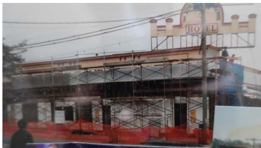
Lifting of new parapet onto the hotel (early 1990s) (Source: Hanging inside Royal Willows Hotel)
