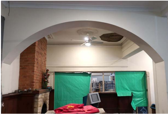
Lath and plaster ceiling to east part of the front room (background) looking south. Modern ceiling to north-west room in foreground
