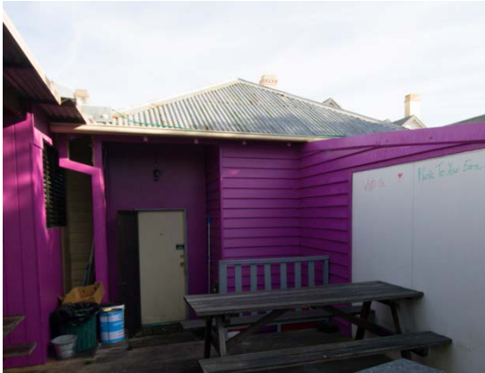
View of hipped roof addition with exposed rafter ends from east (rear) (Source: Gordon Building Design)
